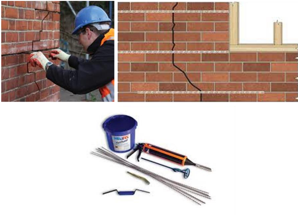
Fig. 9. Strengthenin cracked masonry walls using Stainless steel rods ( https://www.helifix.com.au/ )
