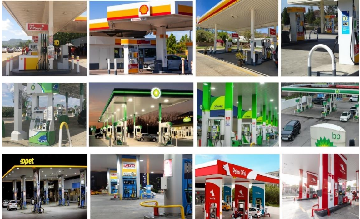
Figure 16 indicates unstandardized and miscellaneous bollard designs and applications at various fuel stations.
