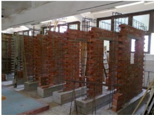
(c) Installation of Bond Beam Reinforcement
