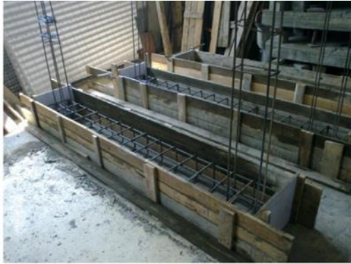
(a) Footing with Column Reinforcement
